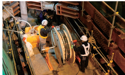
Photo 5 坑内全景 (Panoramic View of Vertical Shaft)
