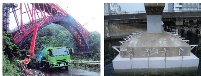
Photo 4 耐震補強工事への適用 (Application for Aseismic Reinforcing Works)
