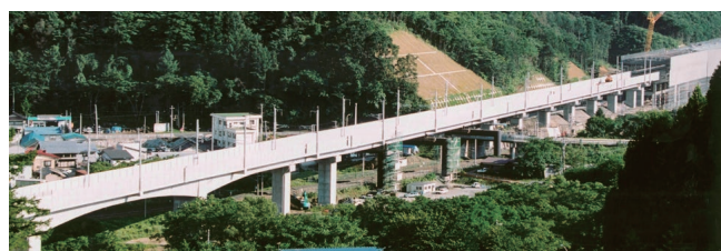
Photo 3 新幹線高架橋への適用 (Application for Construction of Shinkansen Viaduct)
