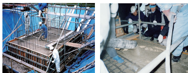
Photo 2 実規模施工実験の状況 (Scene of Construction Tests on Full-scale Members)
