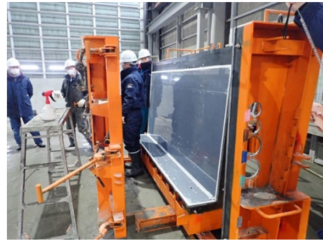
Photo 1 型枠へのシートの貼付状況 (Paste Sheet on Formwork Situation)
