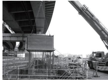
Photo 1 PCa 型枠の建込み (Installation of PCa Formwork)
