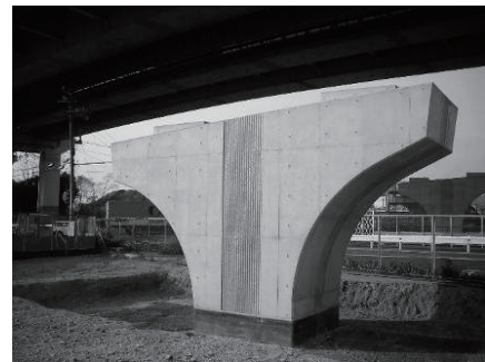
Photo 2 橋脚の施工完了 (Completion of Pier)
