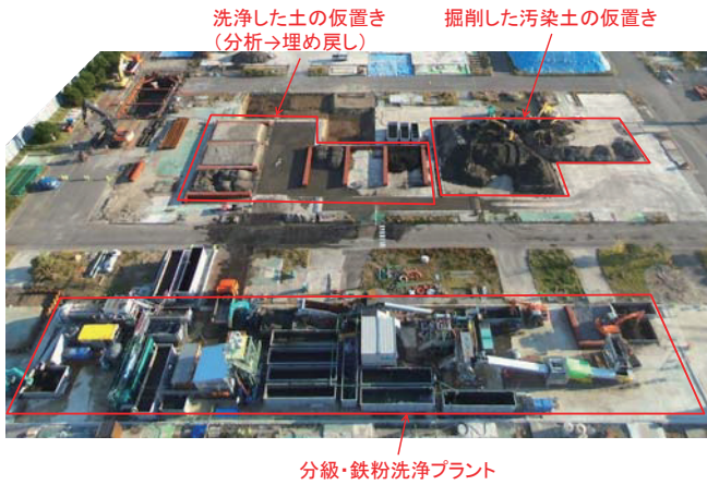
Photo 3 工事中の現場全景 (Panoramic View under Construction)
