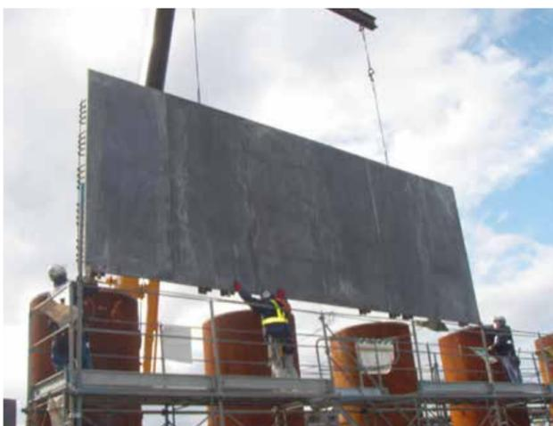
Multiple panels and rebar grid combined into a single large formwork for a wall
