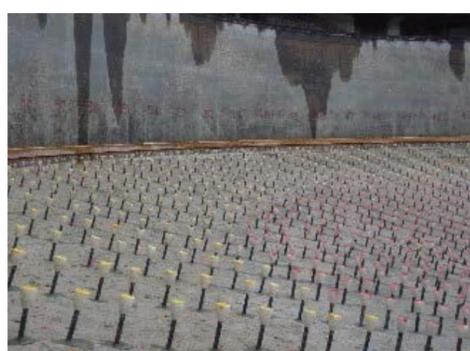
Reinforcement for a bottom plate of the gravity thickening tank
