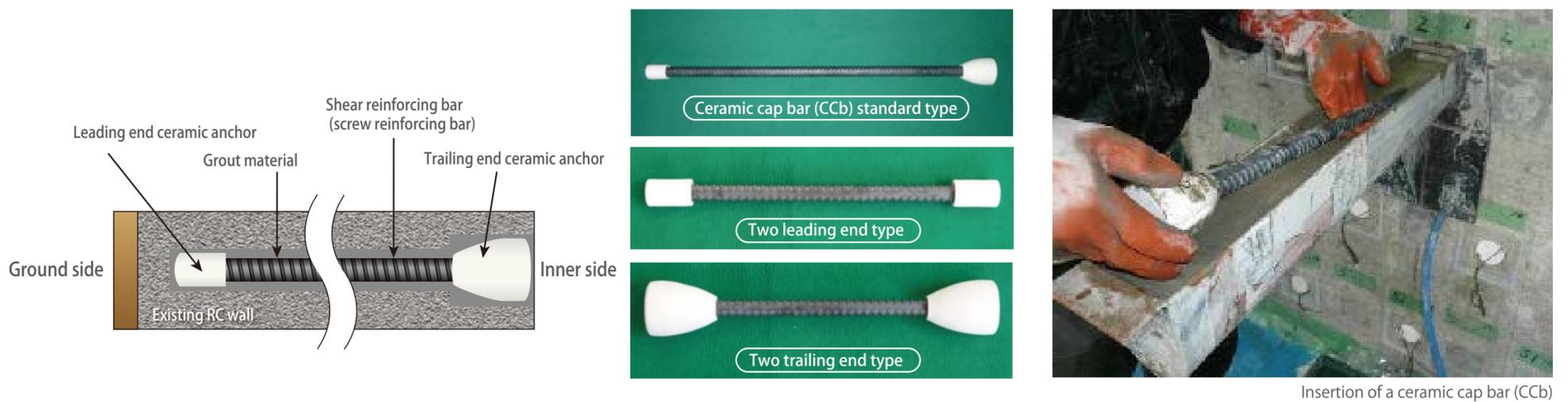
Insertion of a ceramic cap bar (CCb)
