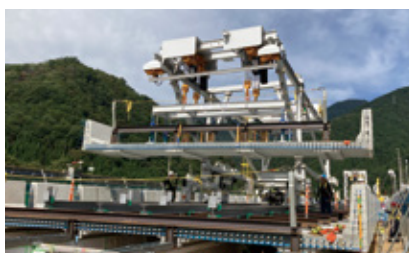
Erecting the new deck for the Anogawa Bridge on the Kan-Etsu Expressway
