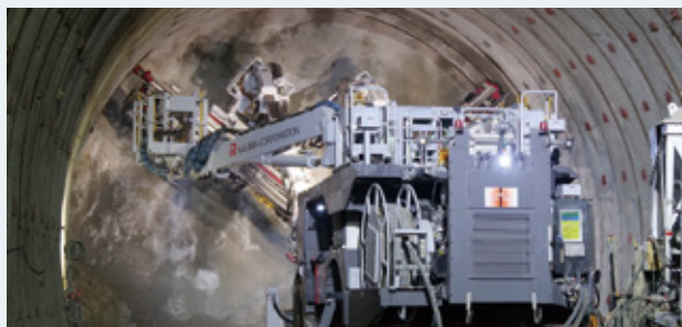
A4CSEL for Tunnel, automated rock bolt installation
