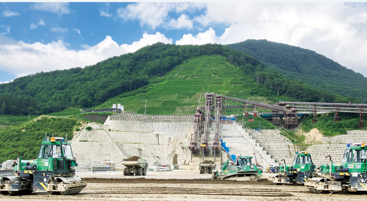
A 4 CSEL*-guided automated construction machinery building an embankment at Naruse Dam (August 2023) * A 4 CSEL: Automated/ Autonomous/ Advanced/ Accelerated Construction system for Safety, Efficiency and Liability
