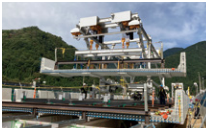
Erecting the new deck for the Anogawa Bridge on the Kan-Etsu Expressway
