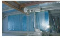
Fireproof coating sprayer robot (smart construction technologies)
