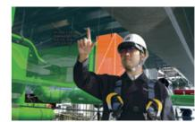
Checking the construction alignment by overlaving the actual product and BIM (BIM utilization)
