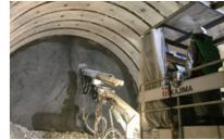
Automation of spraying operation
