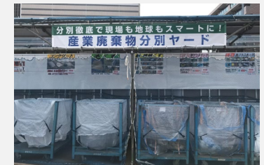
Thorough separation and collection of various types of waste at a construction site sorting area
