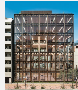
Jutec headquarters building constructed using FR Wood, a laminated pure-wood fire-resistant structural lumber developed by Kajima
