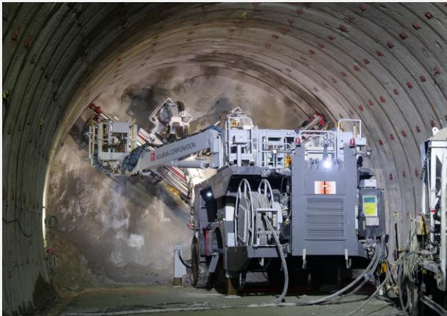
A4CSEL for Tunnel, automated rock bolt installation
